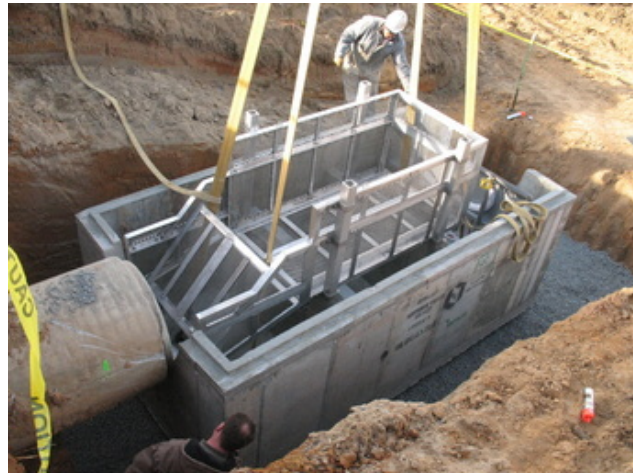
Figure 4.3: Three-chambered baffle box MTD Installed
