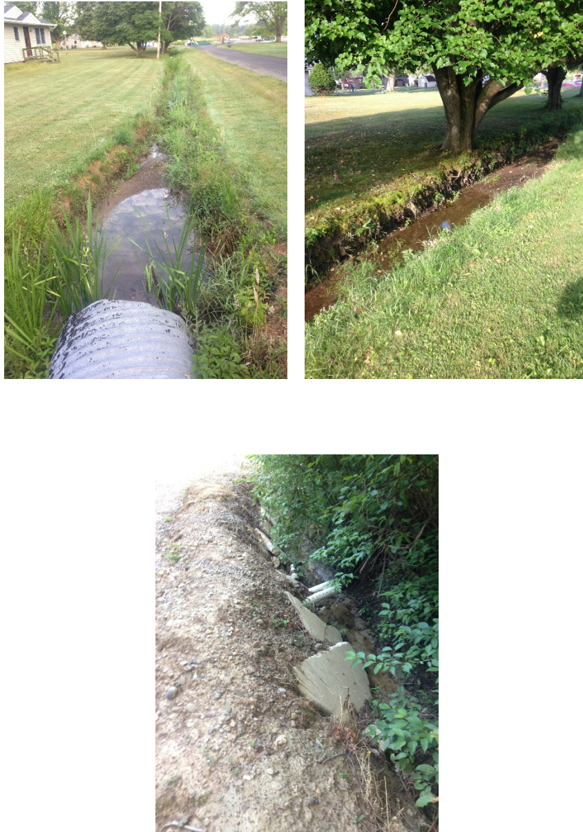
Figure 4.12: Bank conditions at Lauderdale Estates
