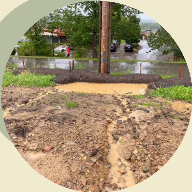
Compost filter sock providing sedimentation control on McAlister's project site
